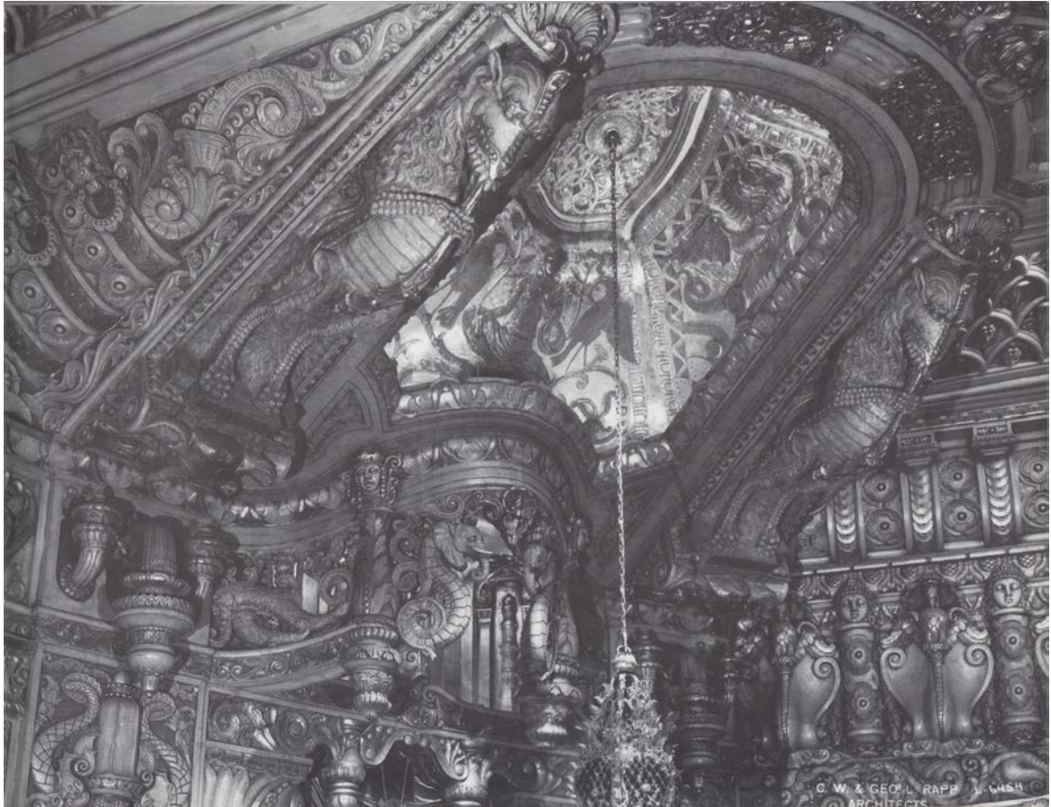
Figure 2.7: These details from the auditorium of the Oriental are rendered entirely in painted plaster. Courtesy Chicago Architectural Photographing Co. Collection, Theatre Historical Society.
